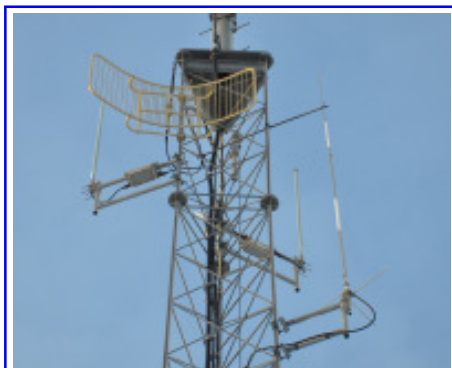
Our FM tower has room to grow.
