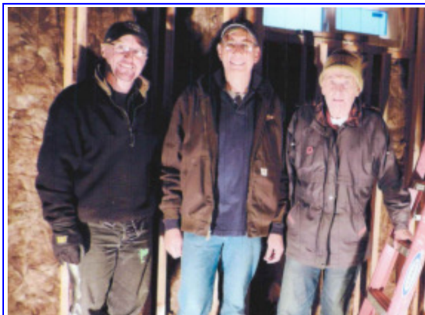
Pastor Michael Coglan, Ron Reckrodt and John Tissell teamed up to install insulation...even under the building.
