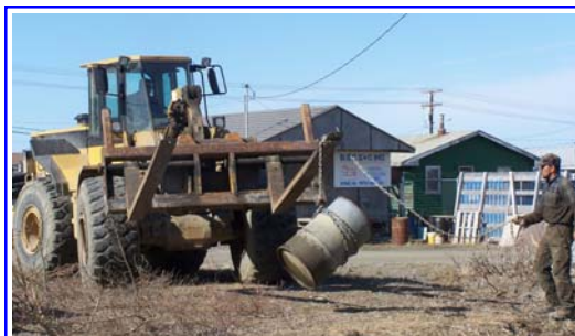
Clearing the site for the new generator building.
