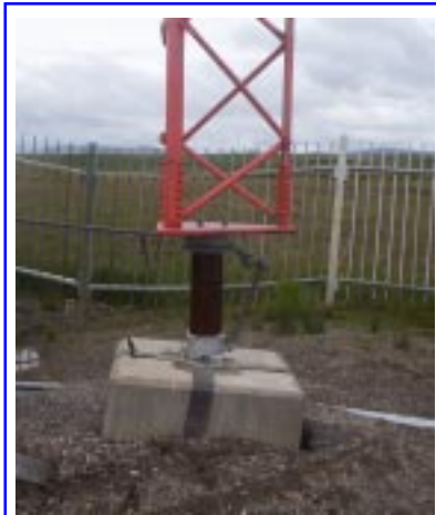
The tilting tower base.
