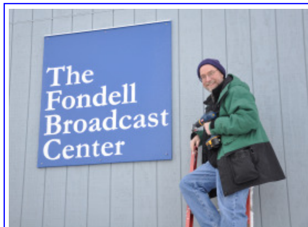
Lon Swanson installing his newest creation.
