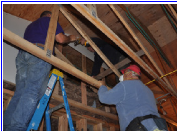
Steve Vonk, Fred Tuggy and Pete Colan wrestle the drywall into the trusses for the firebreak.
