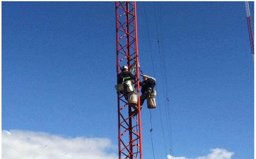
Tower Team replacing braces
