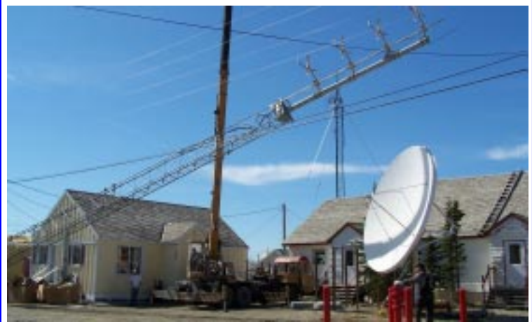
The crane lifts the tower into position.
