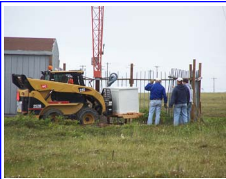
Mounting the West Tower ATU on its new piers.
