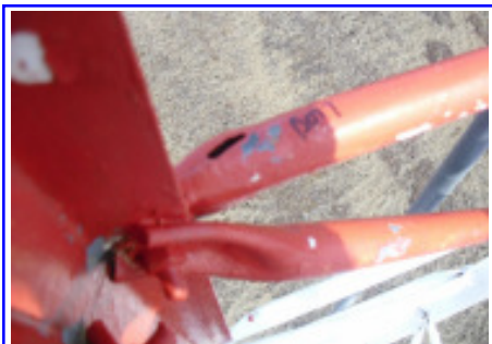
Damaged brackets were discovered on both the East and Center Towers.
