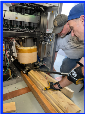
Steve & Nate move the transformer into place in the NX50
