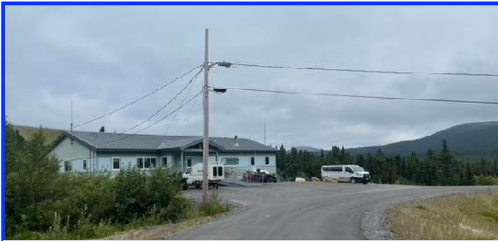
Elim Clinic with the KICY Antenna on the tower on the right of the building
