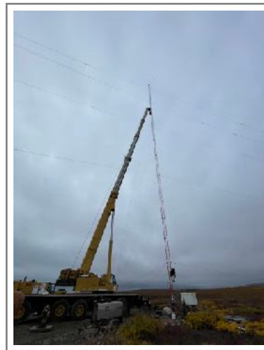
Guy wires are tensioned and a tower guy climbs to disconnect the crane.
