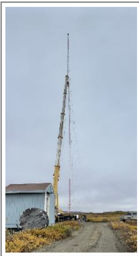
The tower is attached to a crane and the guy wires slacked.
