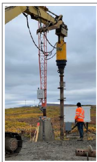
Helicals are drilled into the ground to a depth of 23’.
