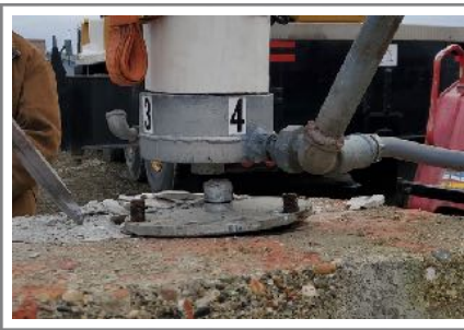
The tower is lifted off the pin it rests on. The old base is push/pulled out of the way and the I-Beam placed on the posts.
