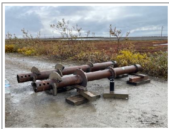
Helical screws for the new base
